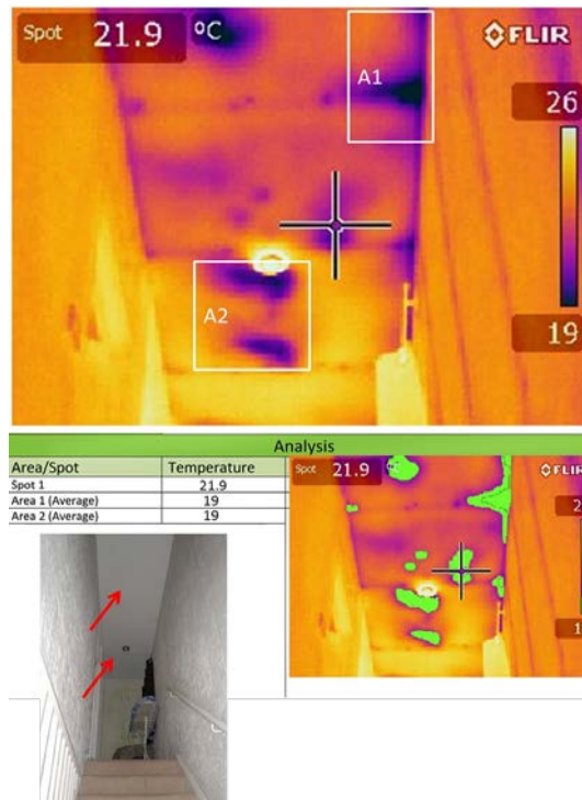
Figure 9: Using thermography for the staircase area
