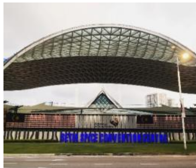
(2) SPICE Roof Structure and Pyramid Skylight
