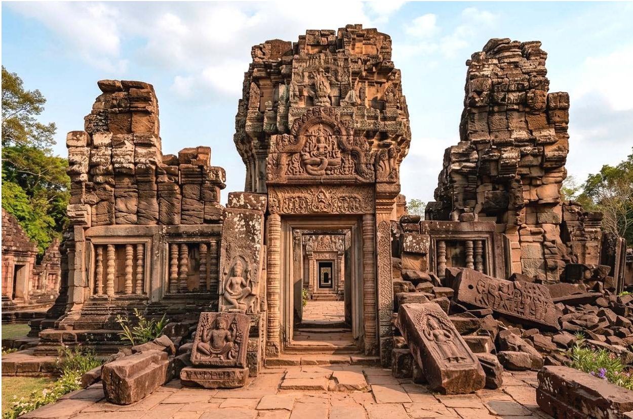
Figure 2: The ruined PHP before the restoration. (digitally remastered image).
